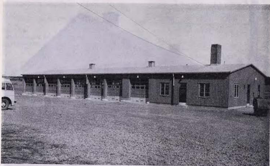
Kungälv's Ytterby, garage.
